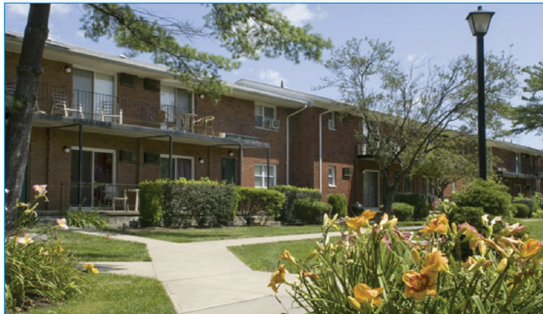
Troy Hills Village, a 752-apartment community with about 1,500 residents, overhauled its HVAC system with new condensing gas boilers, premium pumps and VFDs. Insulation was added to more than 21,000 feet of hot water pipes across the community.
